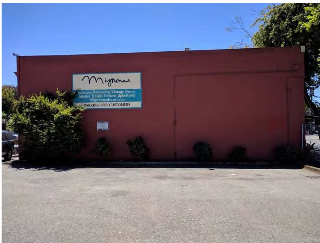
Photo # 4. View of the south Property border and adjoining furniture store.
