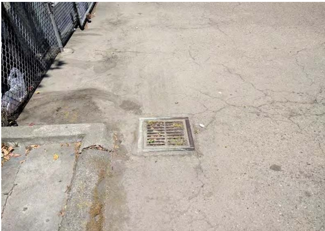
Photo # 6. Surface drain located in the southwest Property corner
